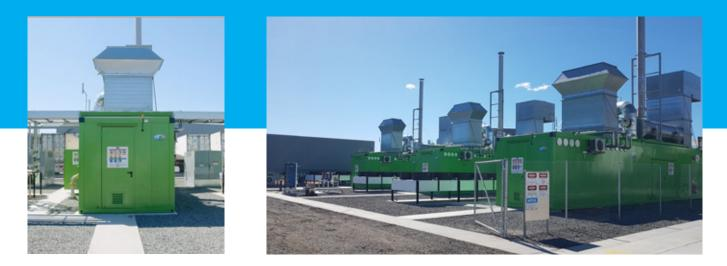
In total, 3 CHP units totalling 4000kW were installed and convert waste product to renewable energy. This project also included the supply and delivery of a turnkey biogas treatment plant including: TS biological scrubber, 2 biogas blowers, 1500kg active carbon filter tank, biogas analyser and heat pumps for scrubber temp control and gas chilling.
